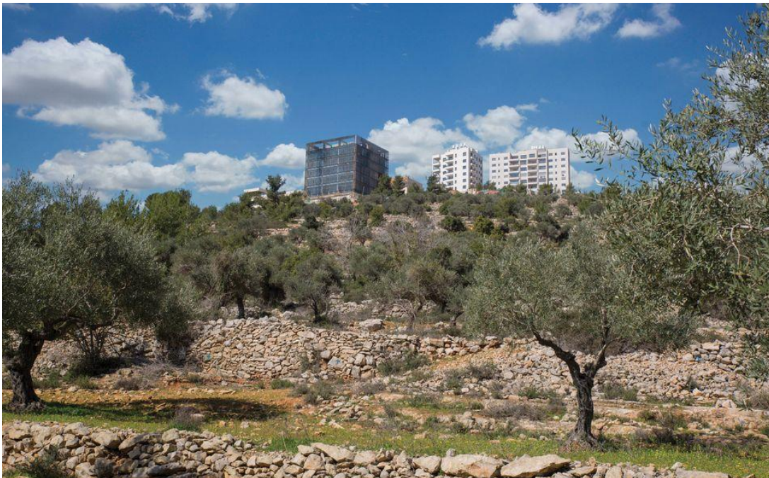
Figure 4. The A.M. Qattan Foundation Cultural Center, set up on a mountain, is a combination of both traditional and contemporary architecture. The Art Newspaper, 2018.
